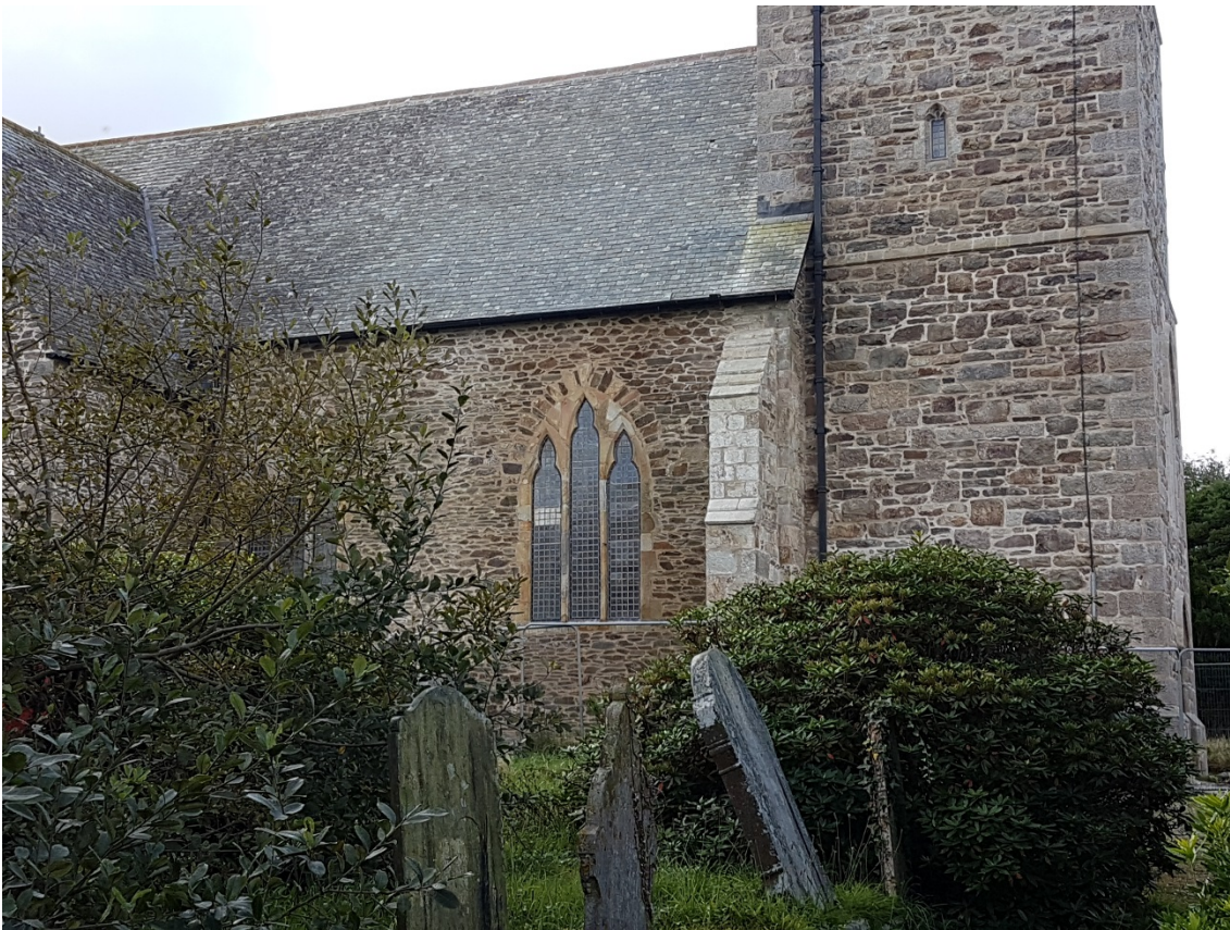
Figure 7 Grade II listed Church of Saint Peter (west facing)
