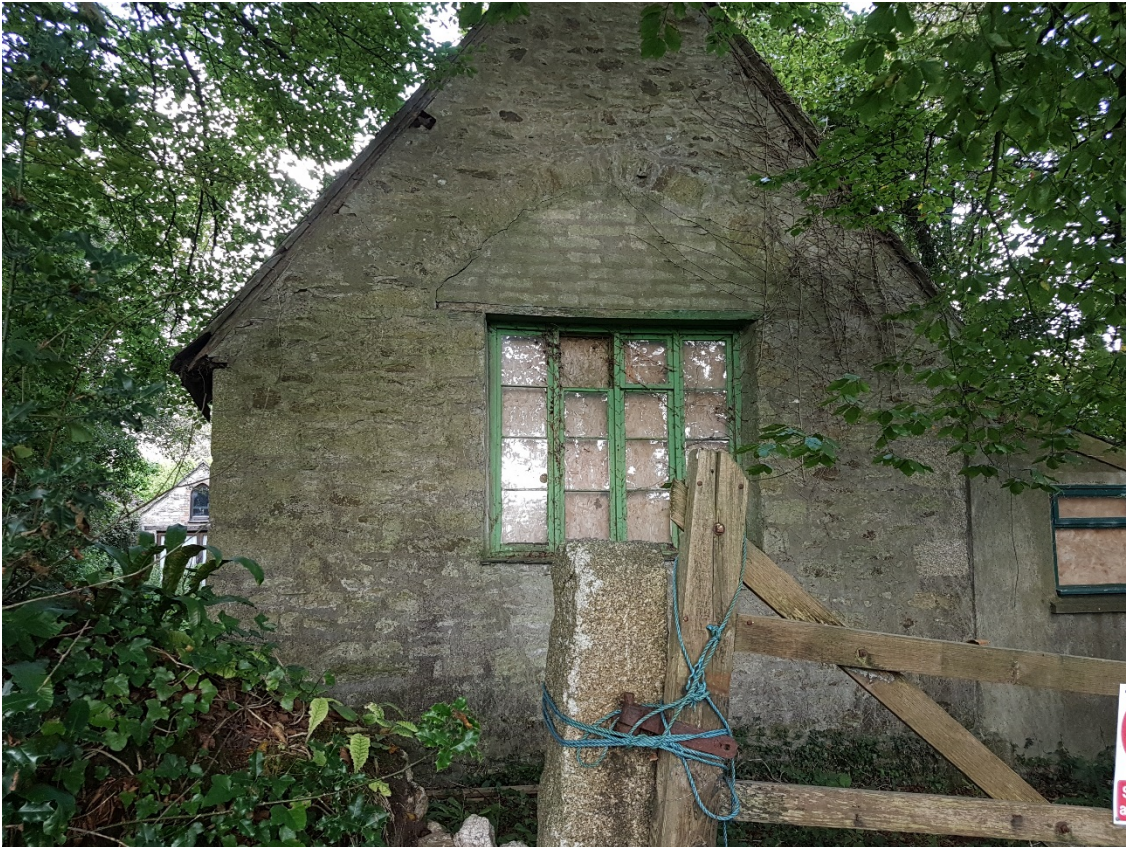
Figure 9 Grade II listed Schoolroom (north facing)
